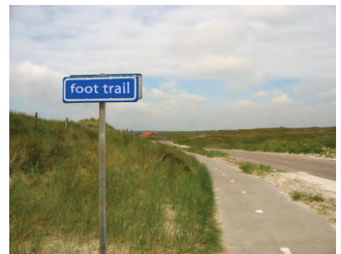
Multi-use trails along rural roadways provide nonmotorized circulation options and can be designed to maintain rural character.
