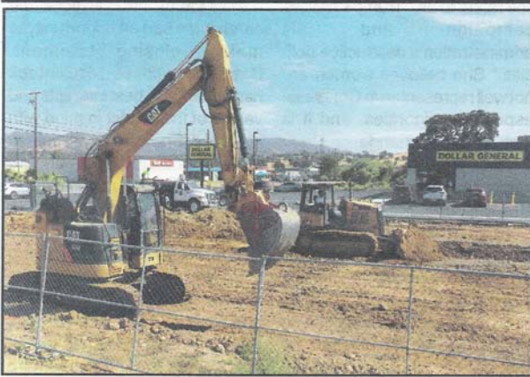
Earthwork has started at the site for AutoZone.
